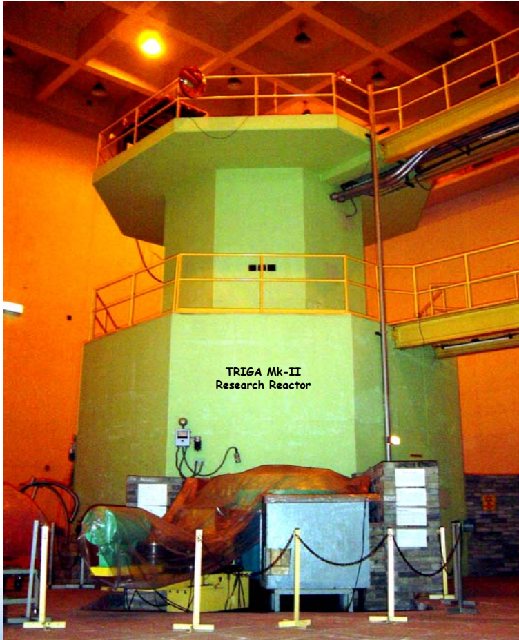
Shield Structure of the TRIGA Reactor
